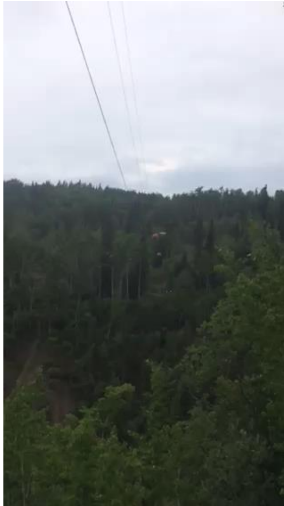
Drone being used to get Strand over Jackass Canyon
